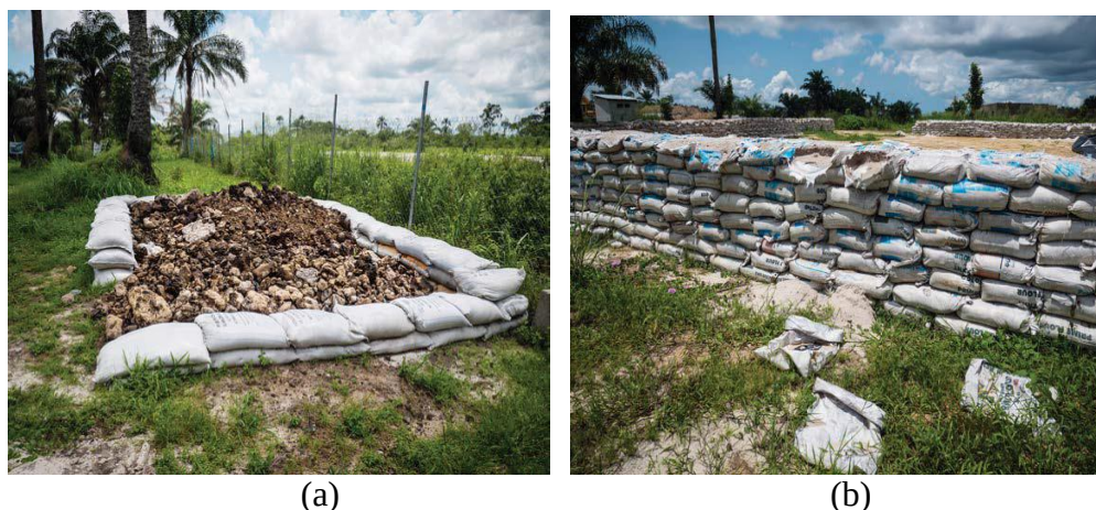
Figure 6: (a) Badly constructed and abandoned Biopile. (b) Incomplete Biopile construction with sandbags used as side walls seen already ripped off, compromising the strength of the biocell wall. Sources: Isaac Harry/cmapping.net, 2020.
